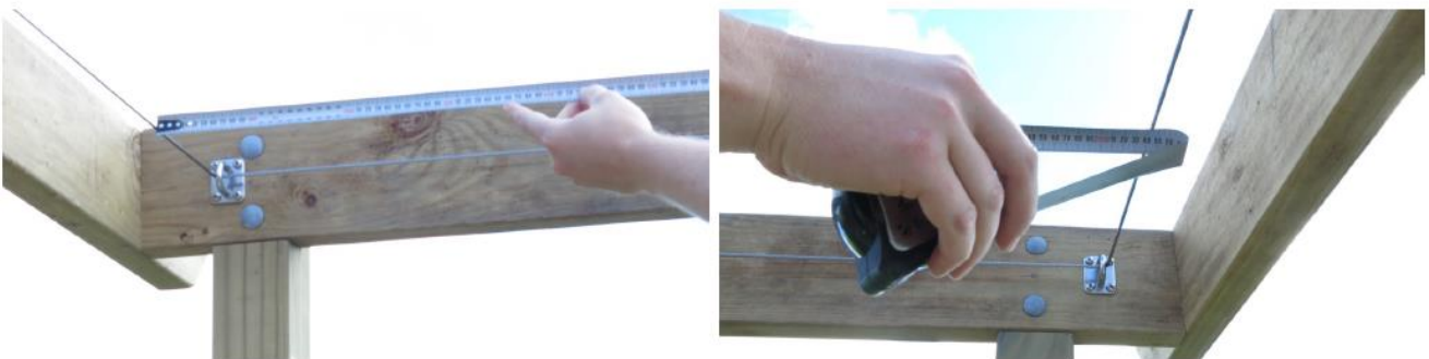
Measure the width between your wire cables, from centre of cable on one side to centre of cable on the other side
